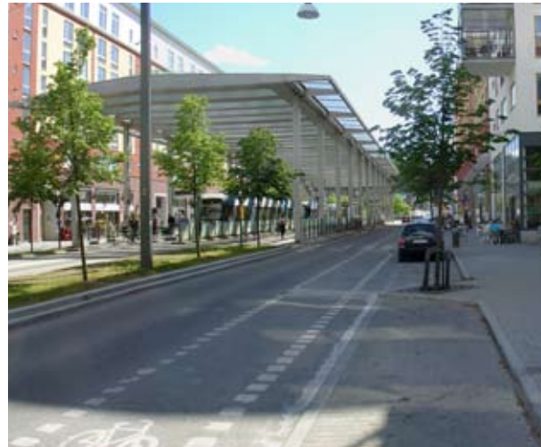
Weather-protected in-street transit stop (Sweden)
